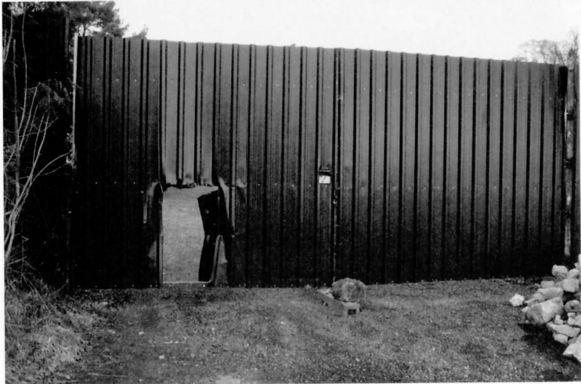
Poorly executed and utilitarian metal gates more akin to a junk yard.
